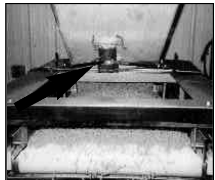
SPR-60 preventing hangups in hopper with pasta feeding weigh belt feeder.
